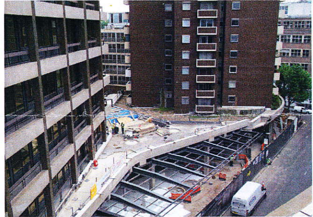
VIEW FROM No.2 STEPHEN STREET
